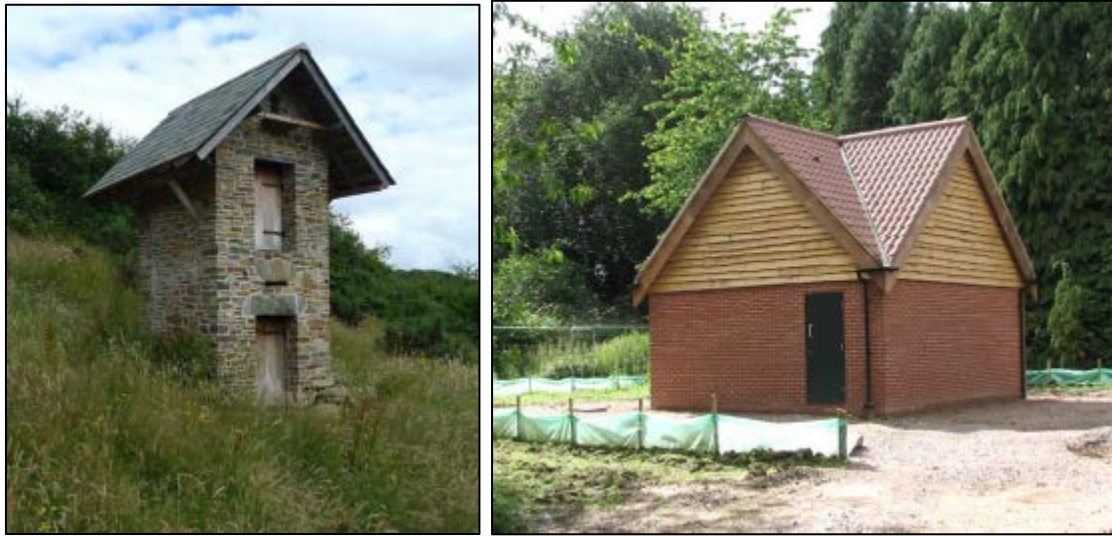
Figure 10. Example of a wildlife tower and waney-edge cladding modifications for bats.
